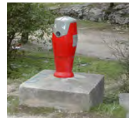
Poteau incendie; Source : Service Forêt
